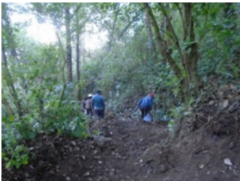
Firebreaking construction, SINERGIAS
